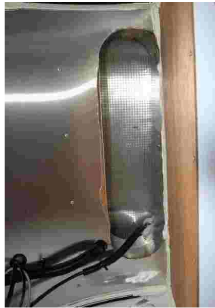
2: PV Panel Wire Through Refrigerator Roof Vent
