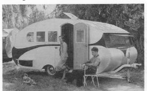
Those first trailers were built of plywood, but adding amenities like chemical toilets, ice boxes, gasoline stoves and water pumps. The trailers began to take on a more "aerodynamic" look as Byam utilized aircraft construction methods in order to lessen wind resistance and improve the strength-to-weight ratio of his trailers.
